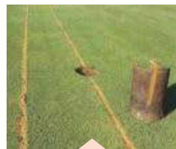
The groove is filled with sand up to 15-22.5cms deep
