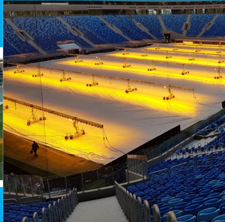
Turf lighting is a necessary reality in stadiums with a covered roof. Lighting units use special light bulbs that have a light spectrum like sunlight, thus replacing sunlight on shaded areas. The growth of the grass and the formation of the root system will be significantly boosted.
